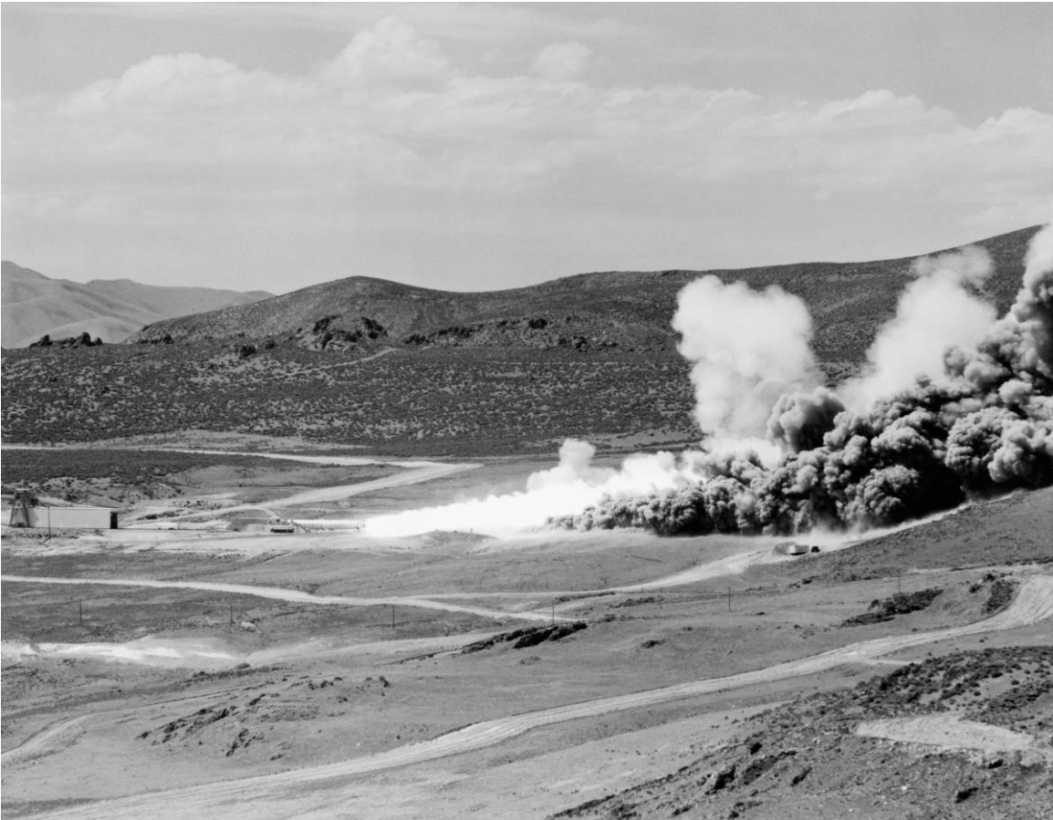
Figure No. E-1. SRB Development Motor-1 (DM-1) in test stand at Morton Thiokol facility at Wasatch, Utah, July 18, 1977.
